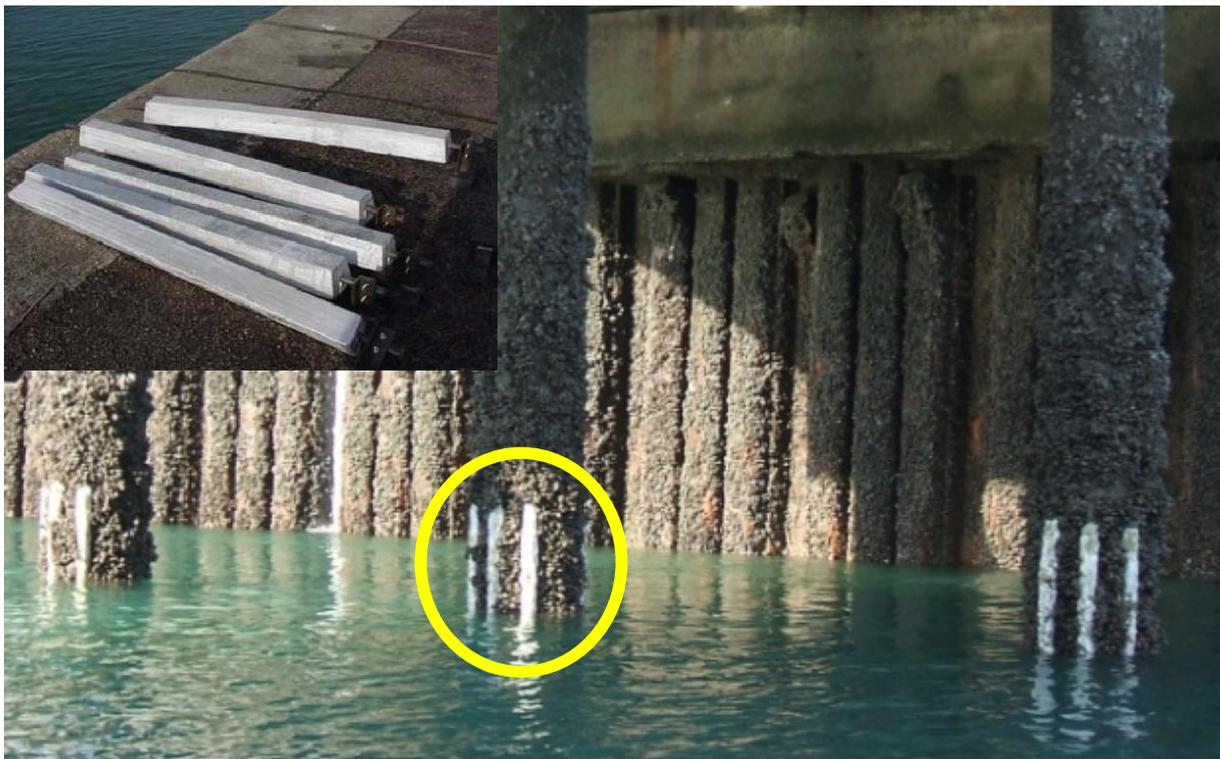
Sacrificial Anodes to protect Port Steel Constructions
