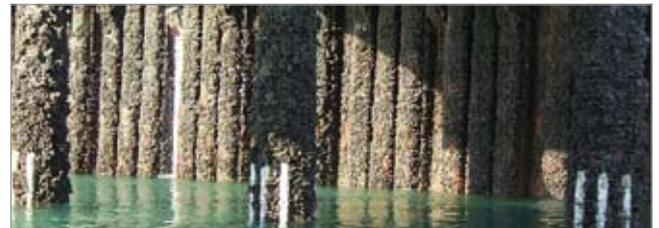
*Visible aluminium anodes on piles (PAH site)*
