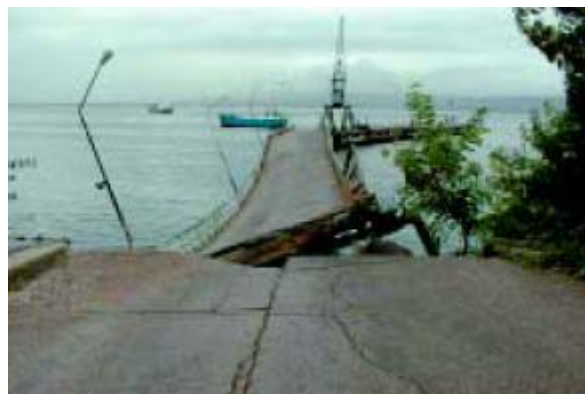
Figure 12: Damage to a bridge to the pier at SEKA paper mill in Izmit
